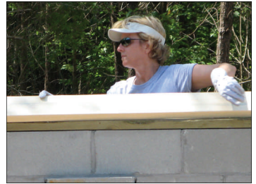
Jody Smith aligns a board for the foundation.
