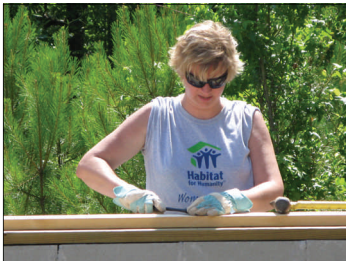
Traci Ellingsworth works on the foundation.
